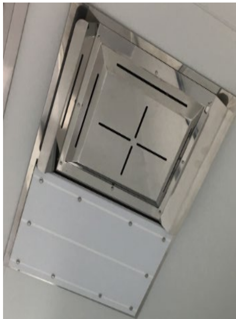
HPG generator & distribution unit
